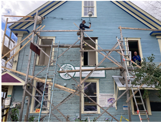
Jason Mallery and Joe John installing windows
