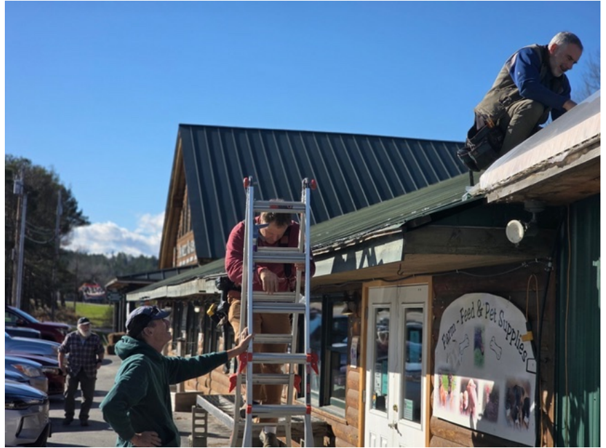
David Ertel, Jeremy Matt and Joe John working on the roof.
